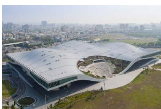
National Kaohsiung Centre for the Arts, Taiwan Size: 141,000 m 2 Year: 2007 - 2018
